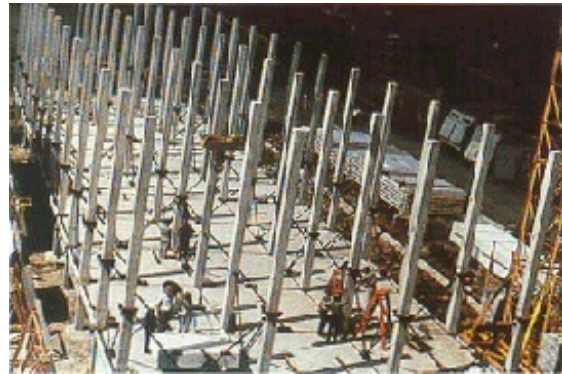
IMS building under construction showing columns under construction
