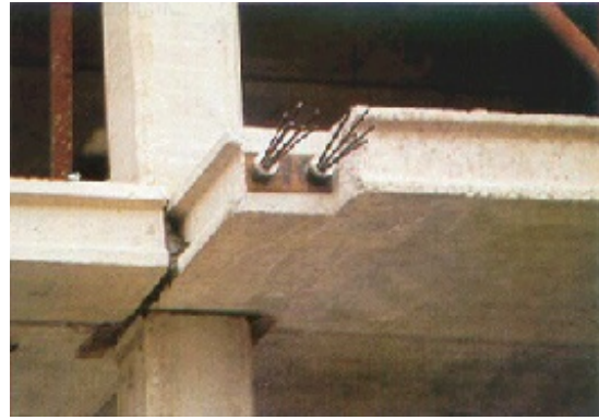
Details of a typical post-tensional slab-column connection
