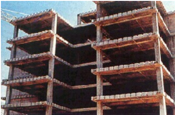
Details of an IMS building under construction showing cantilevered balcony slabs
