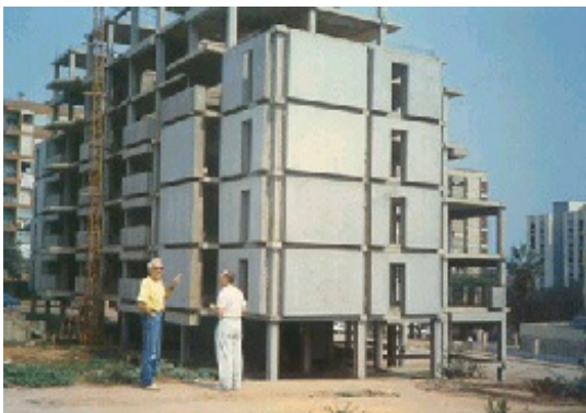
A medium-rise residential building under construction
