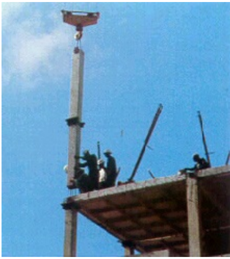
An Illustration of column erection
