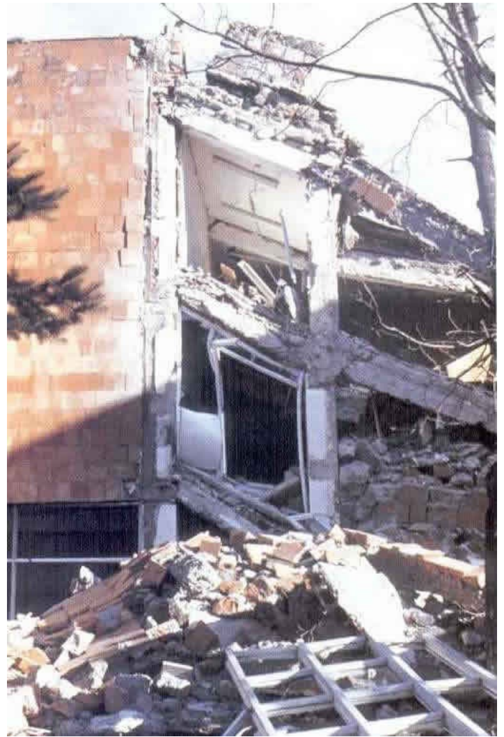
Building Damage (1988 Spitak, Armenia Earthquake) Source: Klyachko 1999
