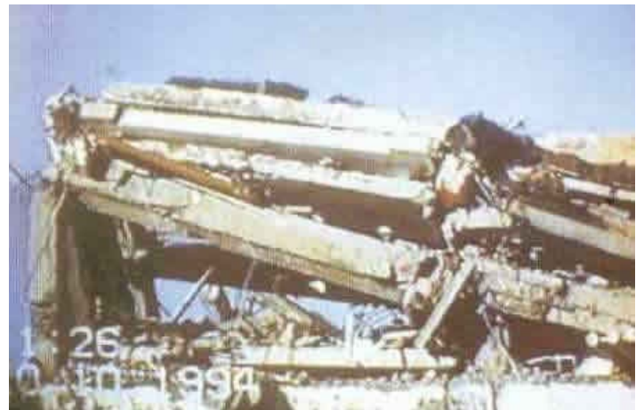
Building Damage (1994 Shikotansk, Russia Earthquake) Source: Klyachko 1999
