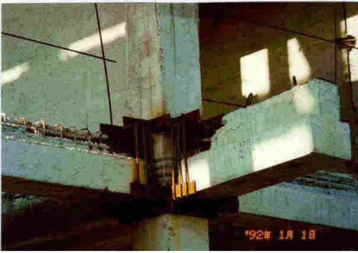
Illustration of Seismic Strengthening Techniques
