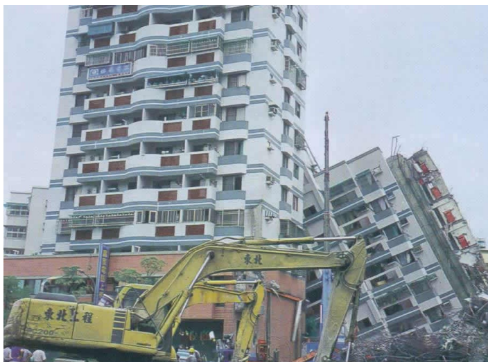
A Photograph Illustrating Typical Earthquake Damage
