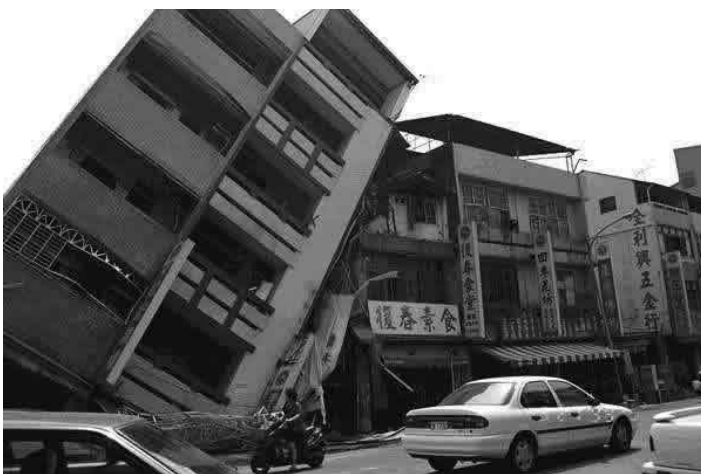
Collapse of a Concrete Frame Building in the 1999 Chi Chi Earthquake (Source: EERI 2001)
