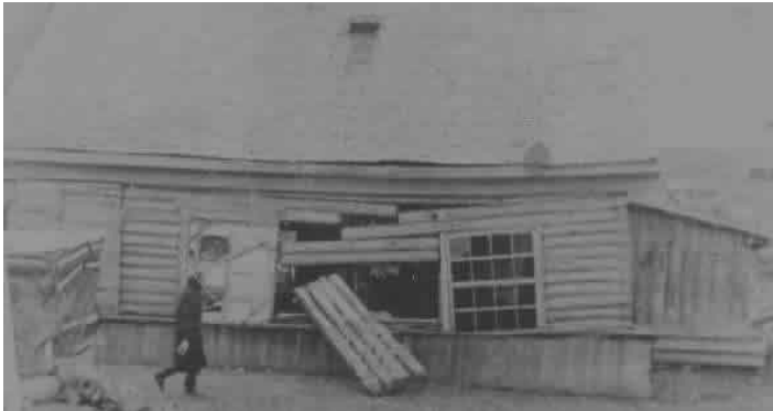
A Photograph Illustrating Typical Earthquake Damage (1958 Kamchatka earthquake)
