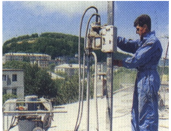
Seismic Strengthening: Application of Post-Tensioning System
