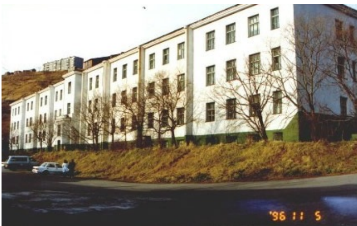
Seismic Strengthening: Application of Post-
