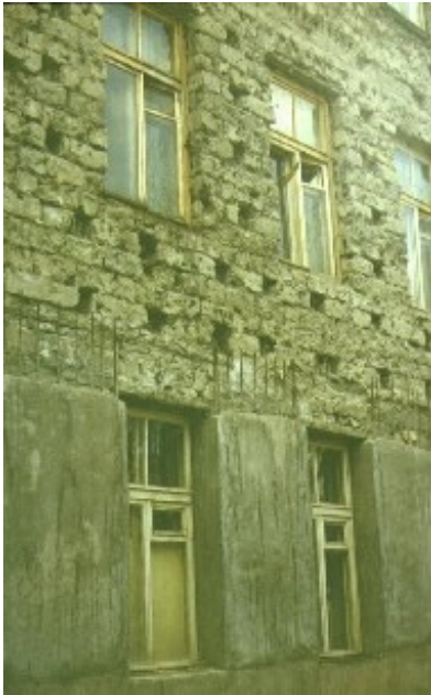
A Building Strengthening Using the Method of Added Stiffness
