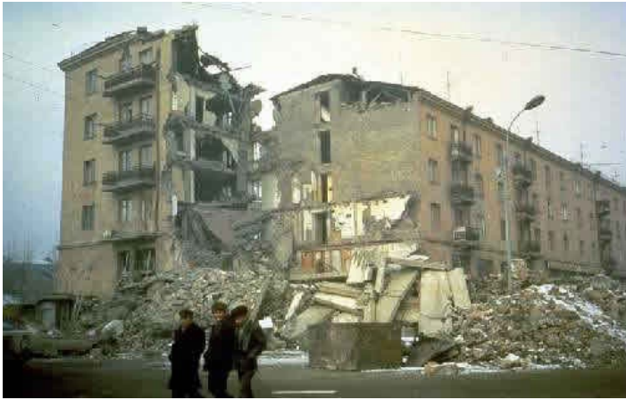
A Photograph Illustrating Typical Earthquake Damage 1988 Spitak, Armenia earthquake Source: EERI
