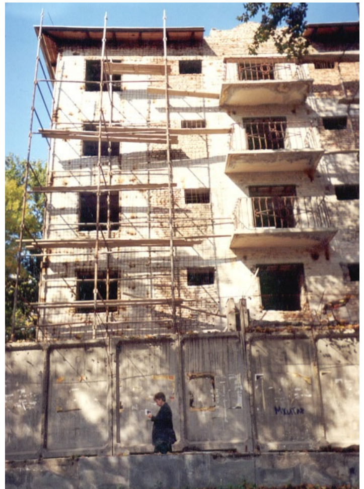
Seismic strengthening under construction
