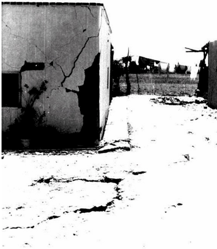
Photograph illustrating typical earthquake damage
