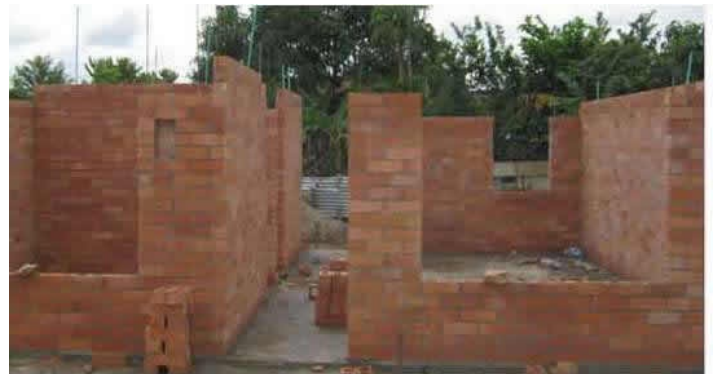
Reinforced masonry walls' assembly after the mat foundation. (August 2011) [1].
