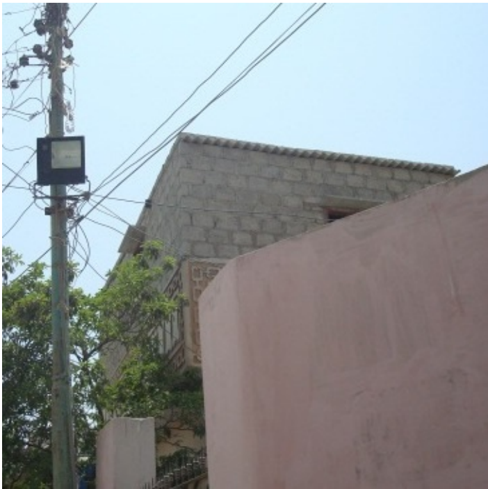
Vertical addition to existing house.
