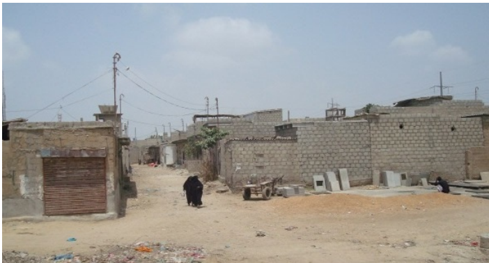
Typical block masonry settlement, Karachi.
