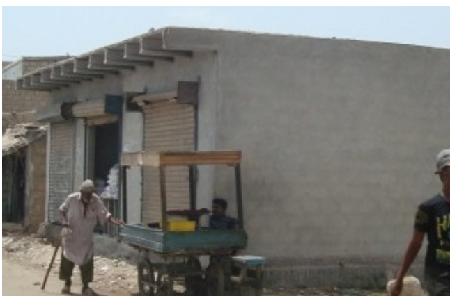
Block masonry with concrete girder roof and concrete tiles.
