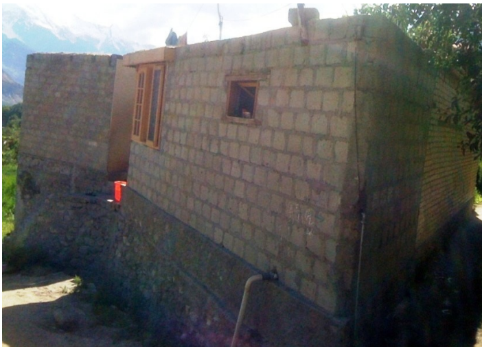
Stone plinth and foundation underneath block masonry.
