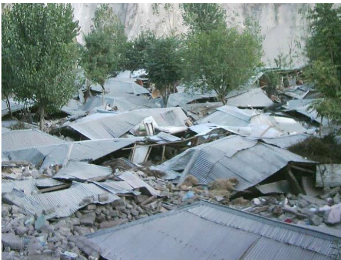
Collapse of unreinforced concrete block masonry houses in Kamsar near Muzaffarabad [5].
