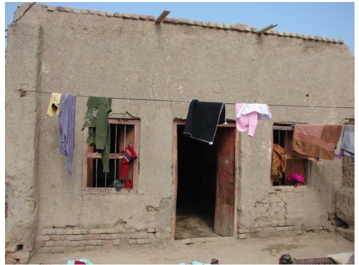
Typical adobe house in Village Vikia Sangi, Larkana.
