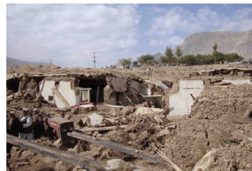
Total collapse of adobe houses during the Ziarat earthquake in 2008.
