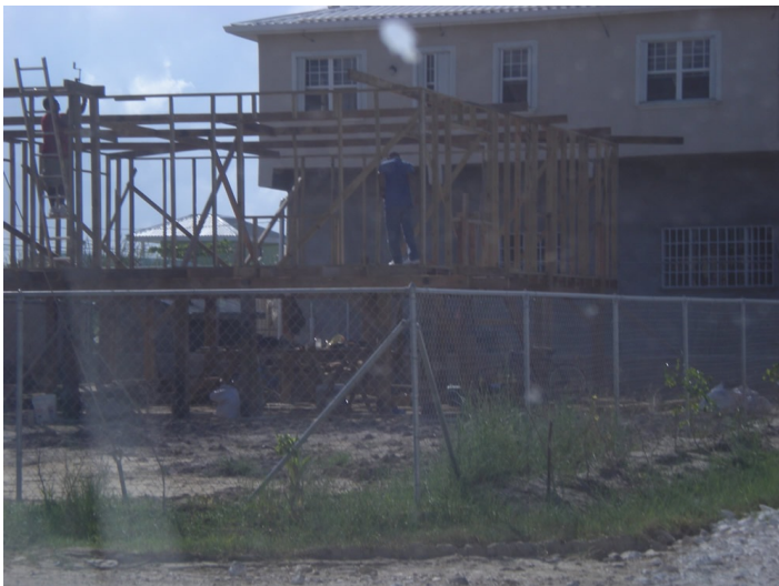
Construction of a timber stilt home
