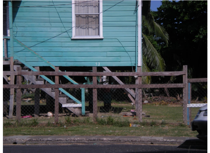
Close up of wood stilts
