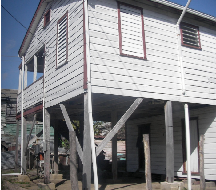
Typical wooden stilt home with a shed added underneath
