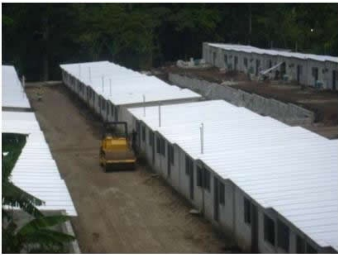
View of several buildings with adjacent walls to neighboring buildings [6].
