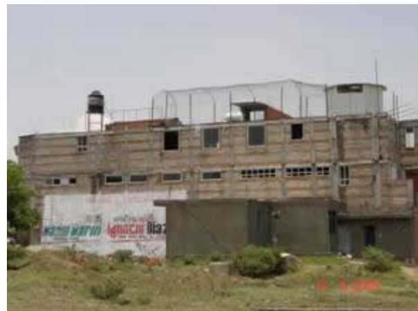
Three-story combined and confined masonry apartment building: 3 courses of bricks alternate with 2 courses of concrete blocks.
