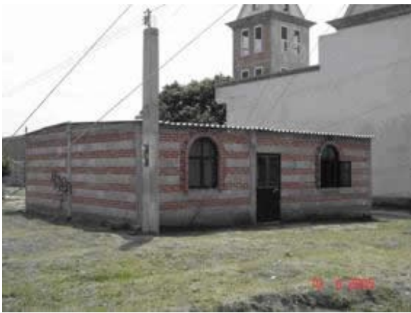
One-story combined and confined masonry house: 3 courses of bricks alternate with 1 course of concrete blocks.
