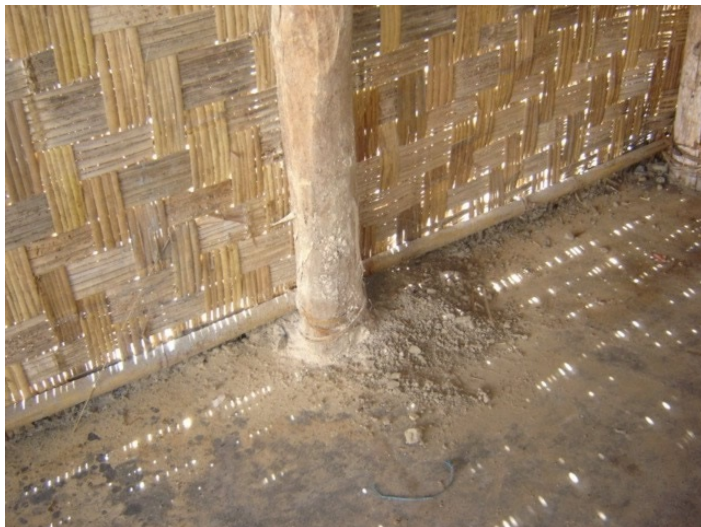
Timber posts are embedded directly into the ground
