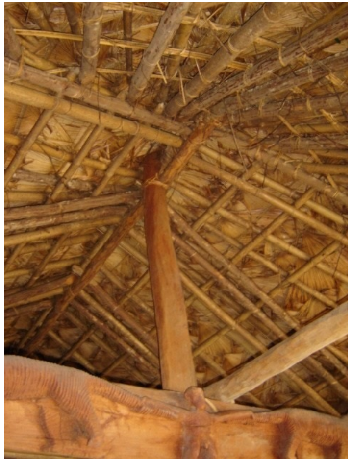
Connection details in the roof understructure
