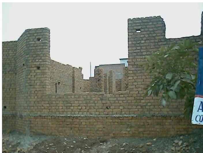
Large openings in walls
