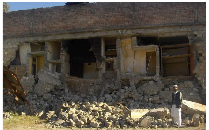
Shinkiari (NWFP Pakistan): out of plane flexural failure of load bearing wall
