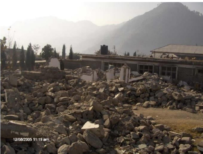
Shinkiari (NWFP Pakistan): out of plane flexural failure of load bearing wall
