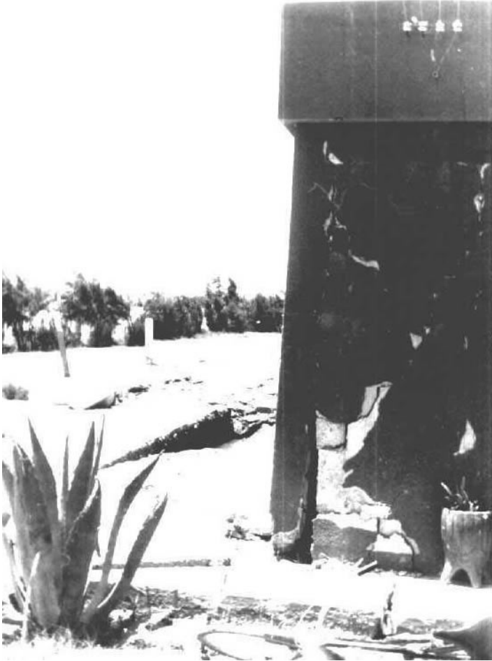
Photograph illustrating typical earthquake damage
